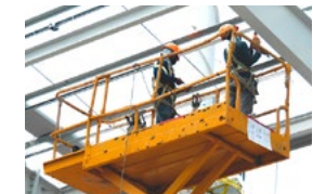
Aerial work platform at construction site
