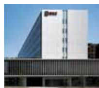
Headquarters / Engineering Research Center
