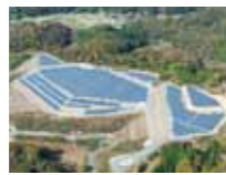
Mega-solar power business
